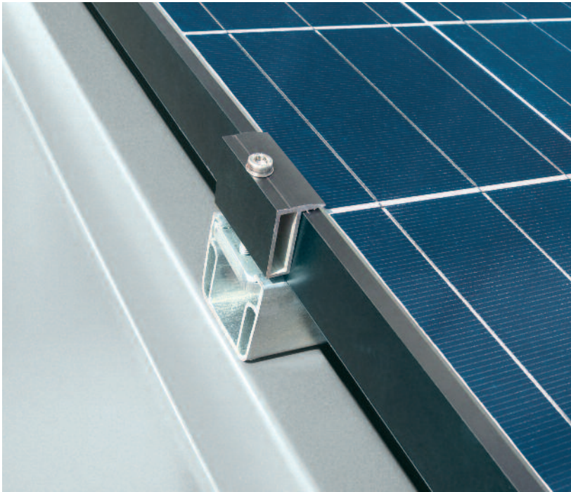
Roof parallel installation on a trapezoidal metal sheet roof
